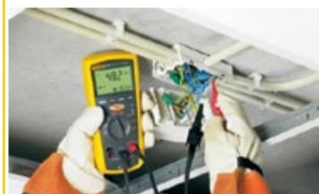
Wiring test in a small distribution box – all in one spot
