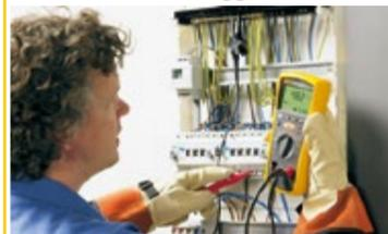
Insulation test at a distribution panel
